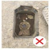
These are **not** acceptable chambers, the hydrant/wash out should be central to the chamber. The cap should always be in place when not in use and the chamber should be clear of any debris. The frame of the chamber lid should rest directly on the top section; no concrete or packing can be used in-between the two.
